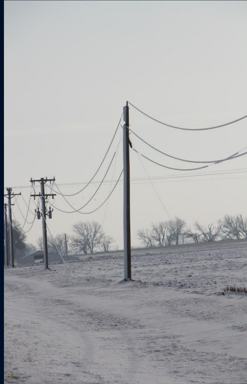
February 25-26, 2013: 'Accretion' damage to Kay Electric Co-op system, Blackwell, OK
